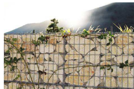
Gabions Crédit photo EDYCEM
